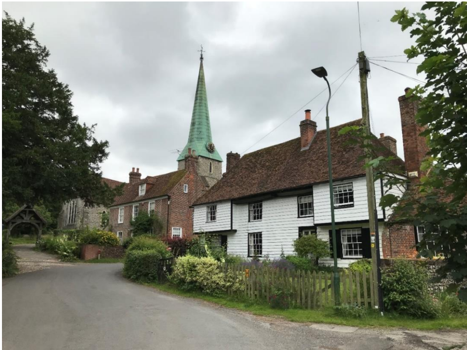
Figure 24: View of Farm Cottage (right), Church Cottage (centre) and St John's Church (behind)
