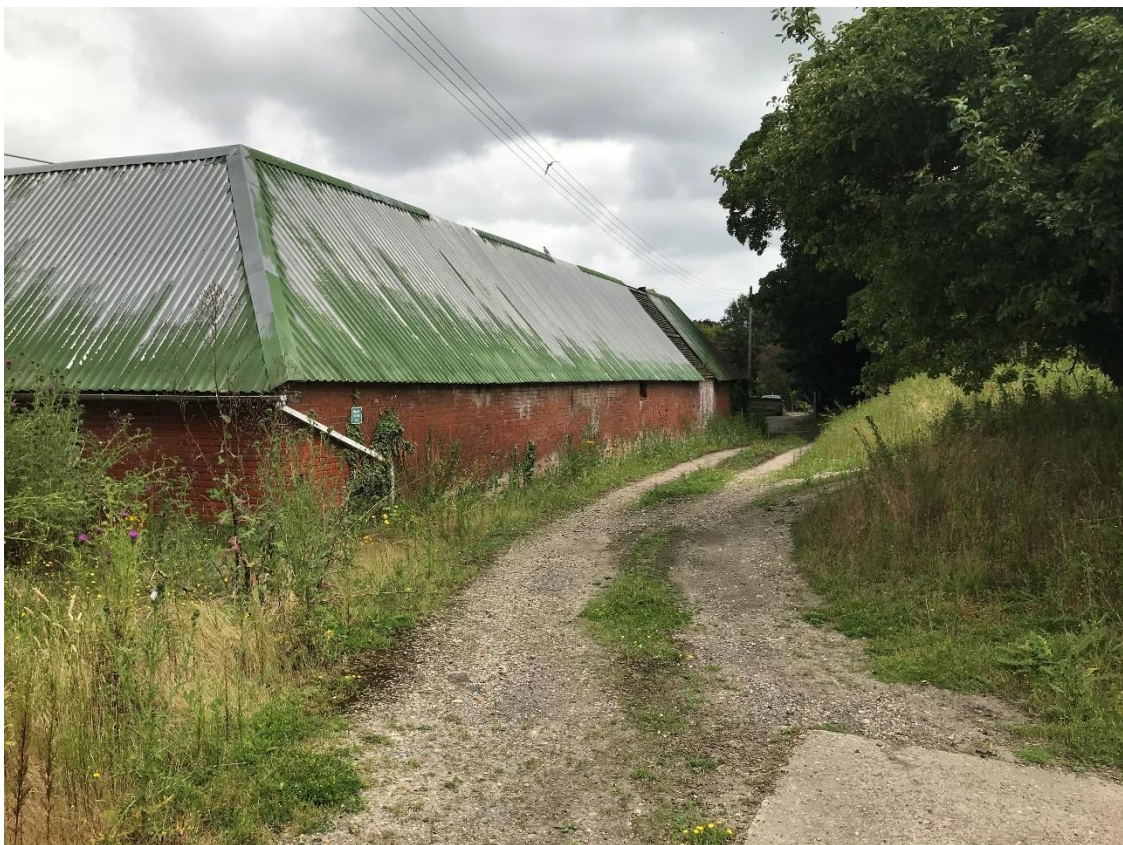
Figure 5: Inter-war livestock range viewed from the south east
