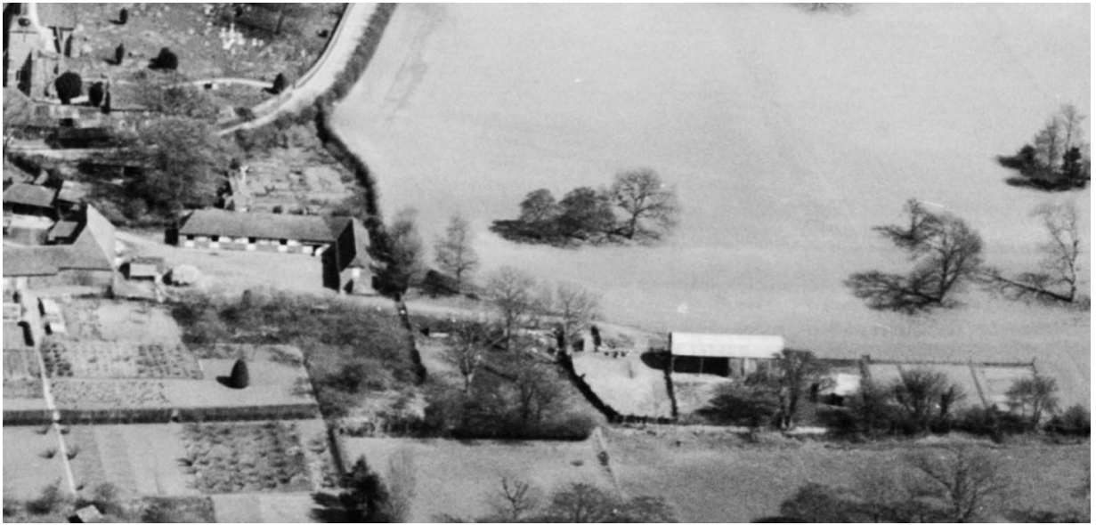
Figure 12: 1947 Aerial View of the Site location from the west. Note the L-shaped range to the centre left of the image, built between 1907 and 1937. Source: Britain from Above website.
