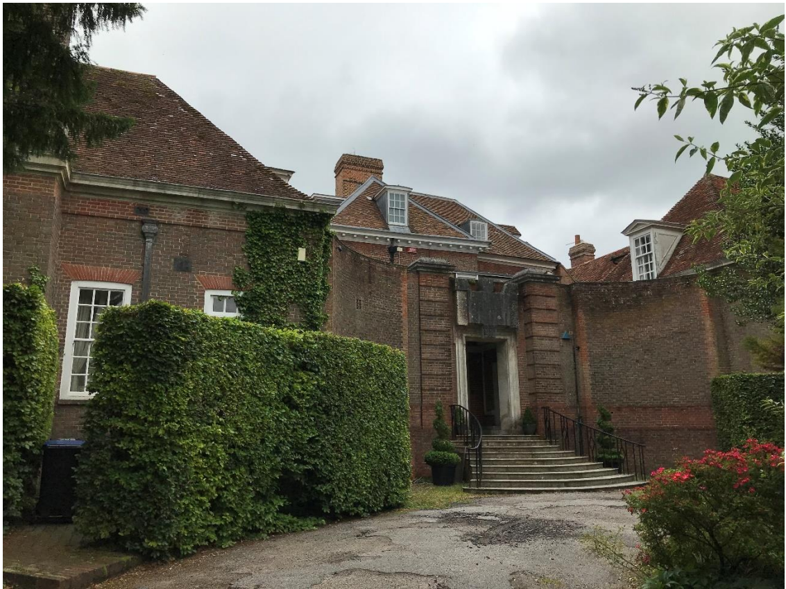
Figure 30: Lutyens' north entrance to Barham Court (1911)
