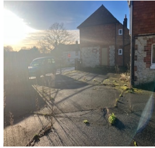
PHOTO 18: Hardstanding and gate to the entrance to the site (east area).
