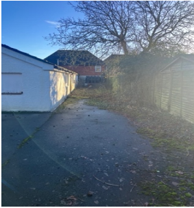
PHOTO 1: West View (back view) of B1 and T1.
