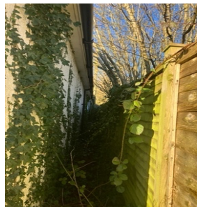
PHOTO 15: North side of the building with common ivy growth and fence.
