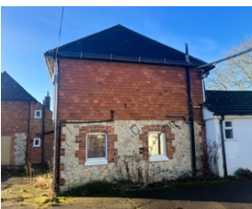
PHOTO 9: North of the building view.
