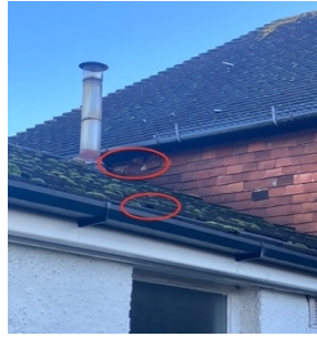
PHOTO 2: B1 gaps (circled) and chimney stack.
