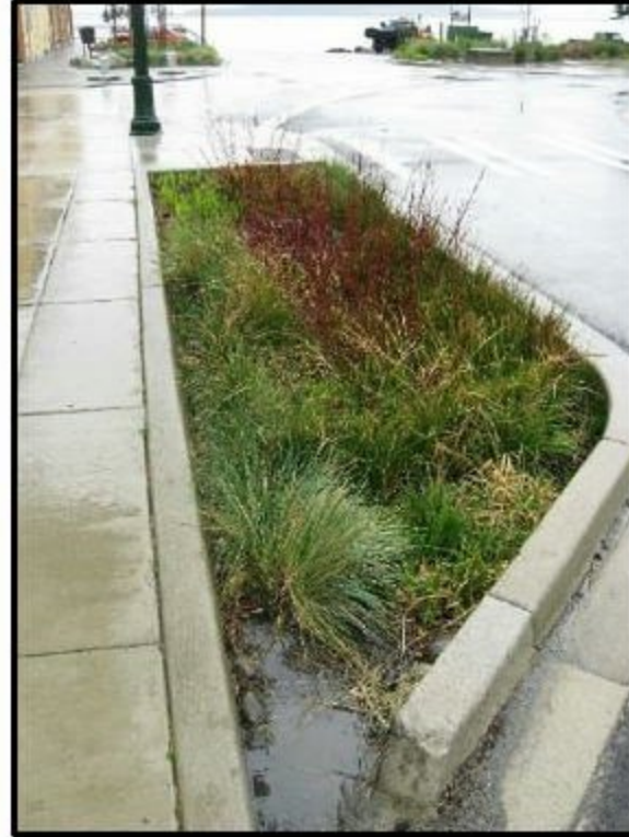
Photo 5.1: Example of a rain garden within hardstanding (Integrity Land Works, 2014).
